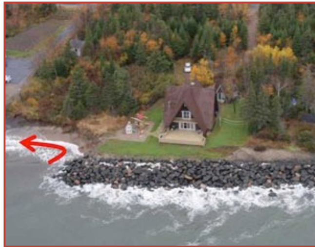
FIGURE 26. Local example of the edge effect in an unconsolidated coast: increased lateral erosion at the down-drift end of a riprap protection structure, Québec North Shore (BERNATCHEZ and FRASER, 2012).
