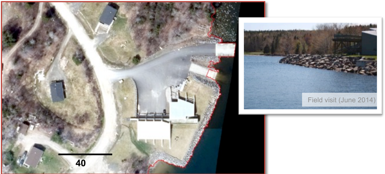
FIGURE 14e. Example of an infrastructure coastline mapped as: CLRIPRAP (red lines). The Feature Codes associated to the different infrastructures begin with the letters “CL”, meaning coastline (as opposed to “SL”, for shoreline ). Even though it exists, the shoreline fronting human infrastructures at the coast is often difficult to identify; the coastline is preferred.
